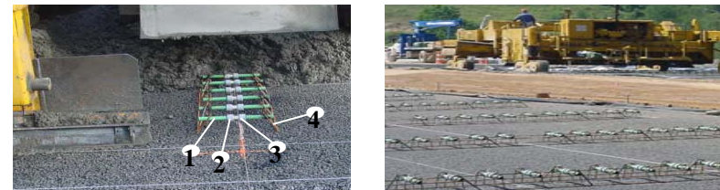
Figure 9. Installation of Modified Dowels on Robert C. Byrd's Highway
